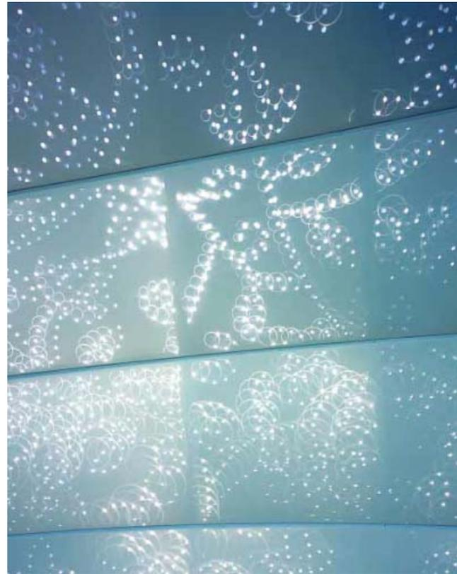
lyweds embrace. Arranged in a looping ivy pattern set into the 11-ton moving wall, 4,700 polycarbonate lenses project light onto a nylon scrim stretched 10 inches from the wall's inside surface. Two hydraulic rams (one at either end) lift the steel veil as if it were a roll-up garage door. "We were concerned about making the whole thing work," says Dytham. "But Kawasaki, who made the rams, said, 'We do stadium roofs that move. This is no big deal.'"
